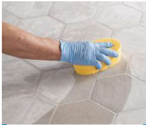
Cleaning and finishing joints with a hard cellulose sponge
