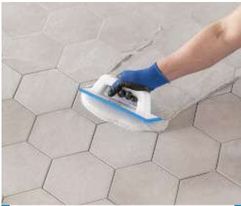
Application of Keracolor FF with MAPEI float
