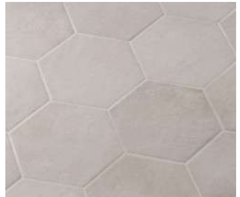
Floor grouted with Keracolor FF
