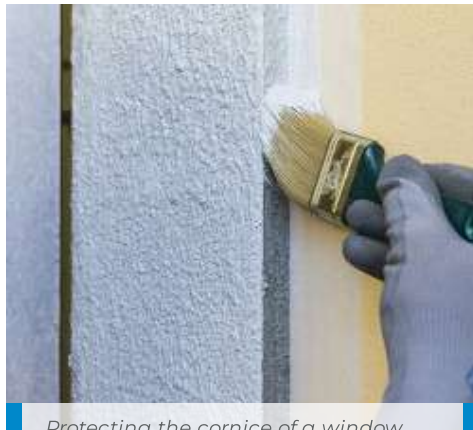
Protecting the cornice of a window with Mape-Antique Ecolastic
