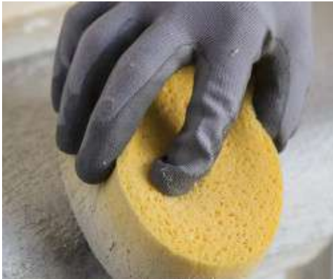
Finishing off Mape-Antique Ecolastic with a sponge float
