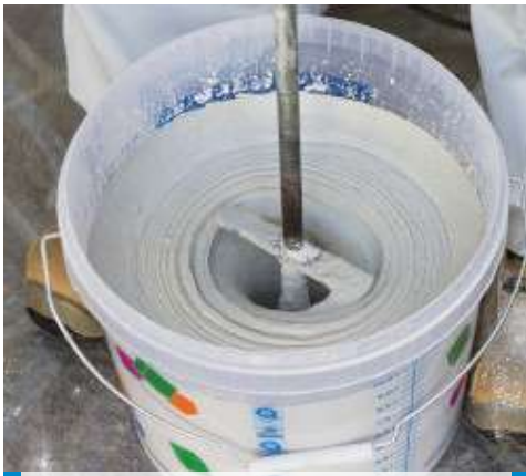
Mixing Mape-Antique Ecolastic
