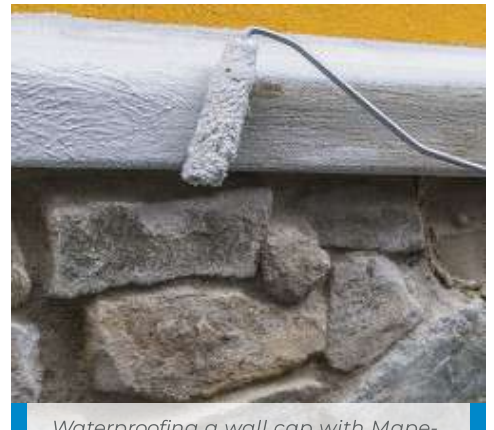
Waterproofing a wall cap with Mape-Antique Ecolastic
