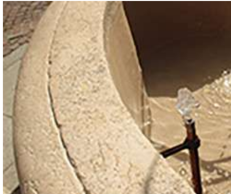
Waterproofing the basin of a stone fountain
